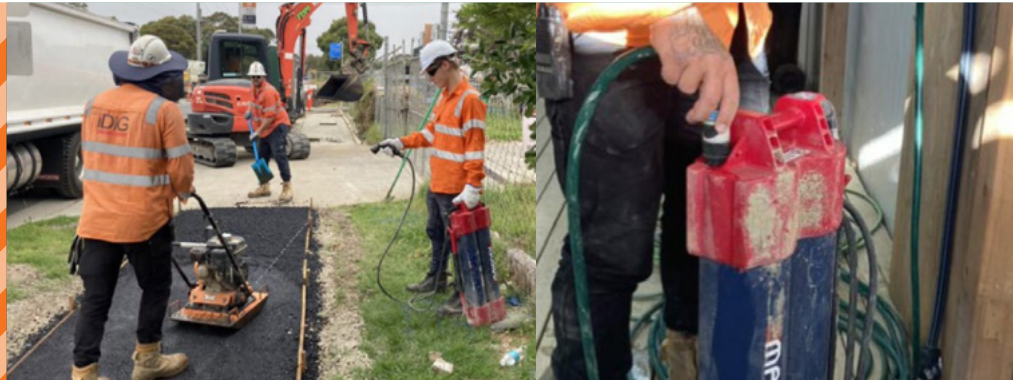
Hose2Go used for asphalt compaction (left), Refilling of the Hose2Go unit (right)
